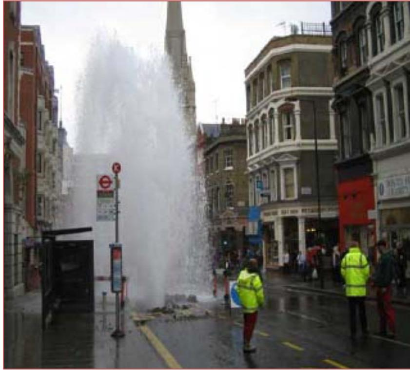
**Most leakage is from distribution pipes - even a big leak causes minimal damage**
